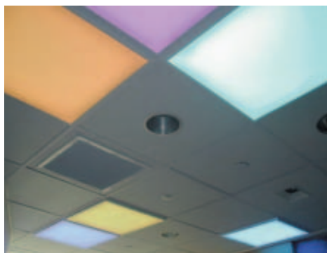
If patients in some rooms in Children's Hospital Boston tire of watching TV, they can stare at the ceiling. Unlike those in most ceilings, the tiles in these rooms light up in a variety of colors from subtle to vivid (courtesy Color Kinetics).
